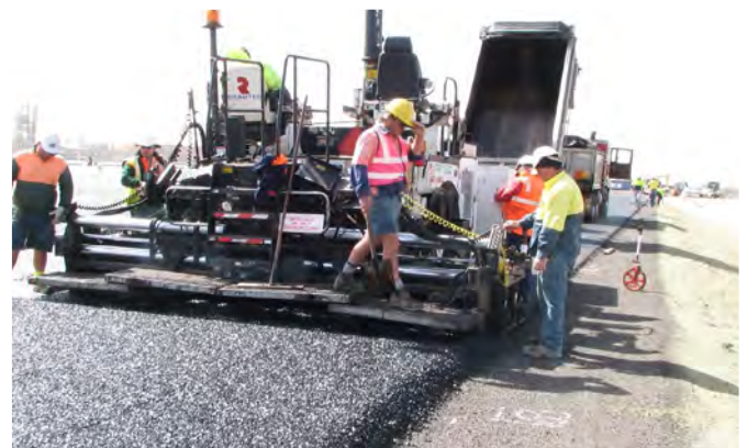
The asphalt carrier mix is applied using conventional paving equipment.
