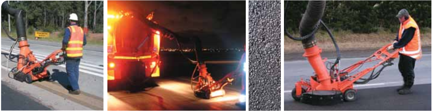
The UHP Watercutter extends the service life of spray seals and pavements. It can be effectively used for line removal (left), airport rubber removal (centre) and pavement rehabilitation (far right).
